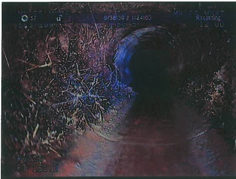
Figure ES - 3 CCTV Results (Root Intrusion)
