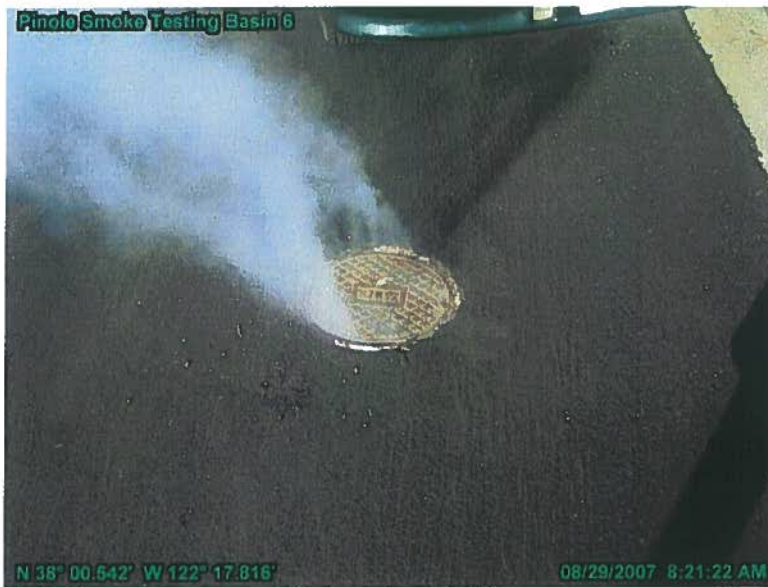
Figure ES - 4 Smoke Testing – Manhole If smoke can get out, then rain can get in.
