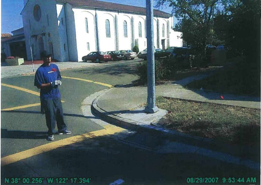
Pinole Smoke Testing Basin 6 Defect 28 - Tennent & Plum - Storm Drain
