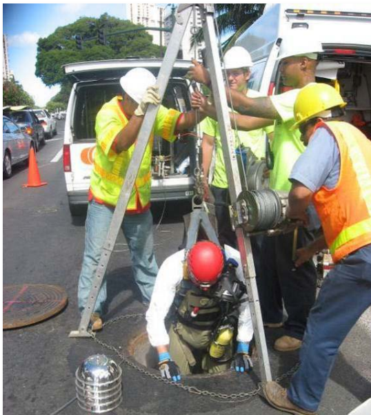
Photo 2-1. Confined Space Entry
